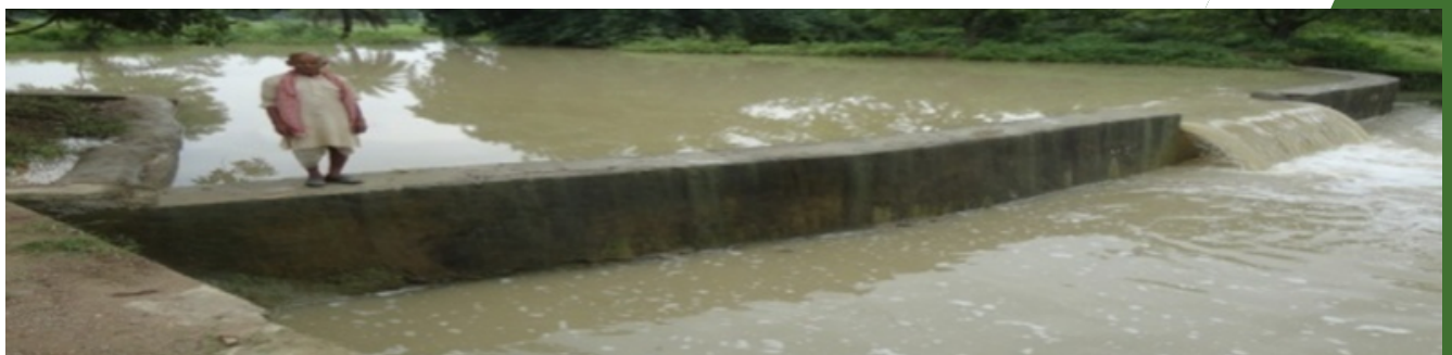
Check-dam water harvesting and storage
